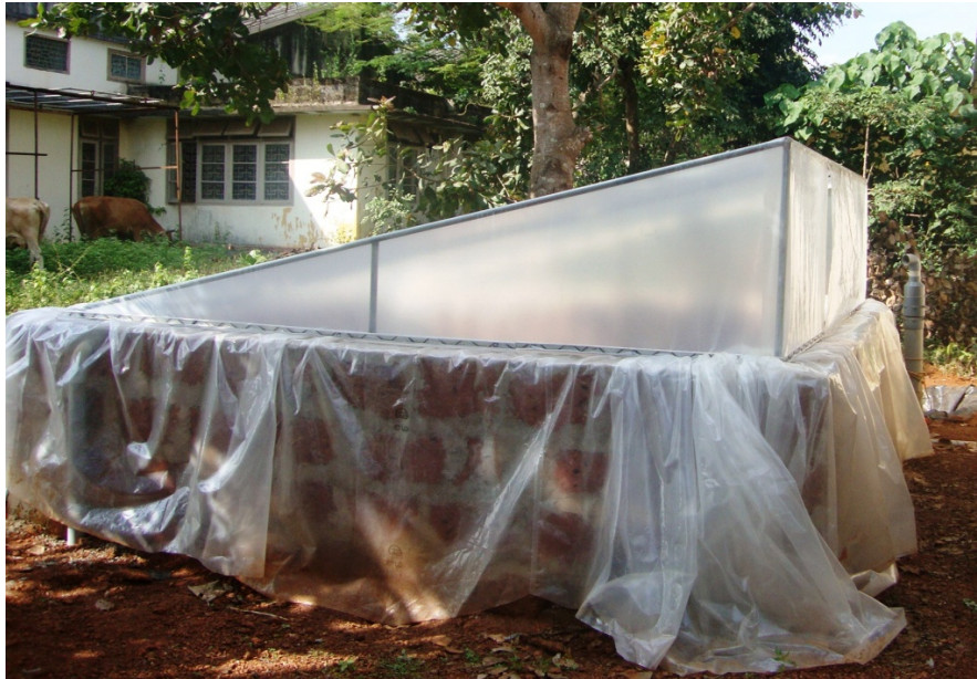
Plate 4.1 Shed roof covered with UVA clear sheet
