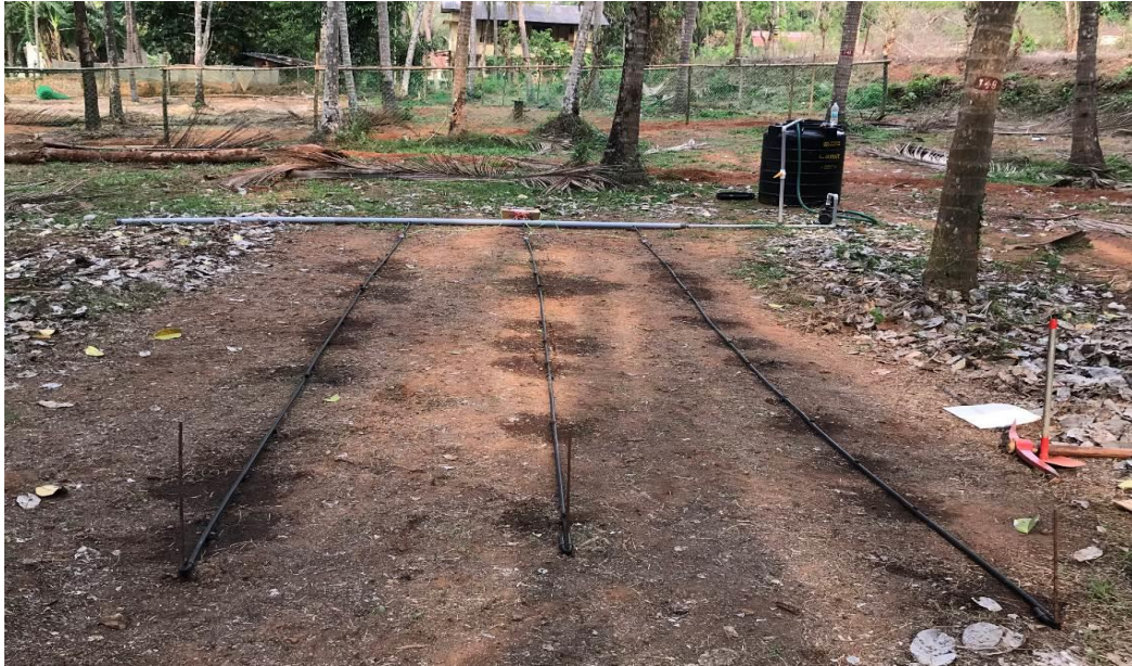
Plate 3.19 Setup for Automated Pulse Drip Irrigation System
