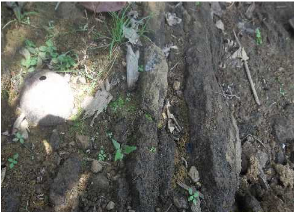
Plate 6. Hard rock exposed at Valarad area
