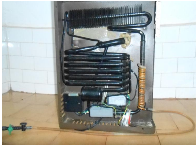
Figure 3.4 Setup for the performance of VARS using hot water from solar flat plate collector
