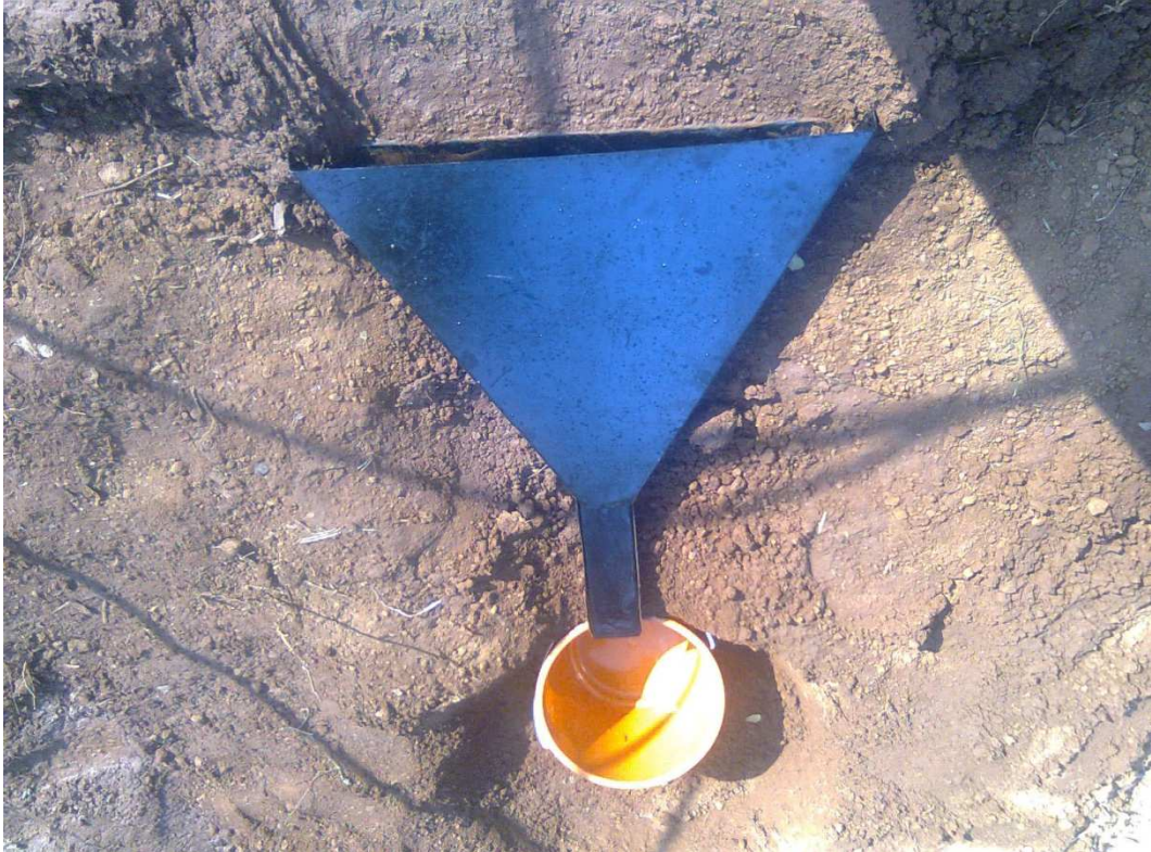
Plate 9. Runoff and sediment collection unit
