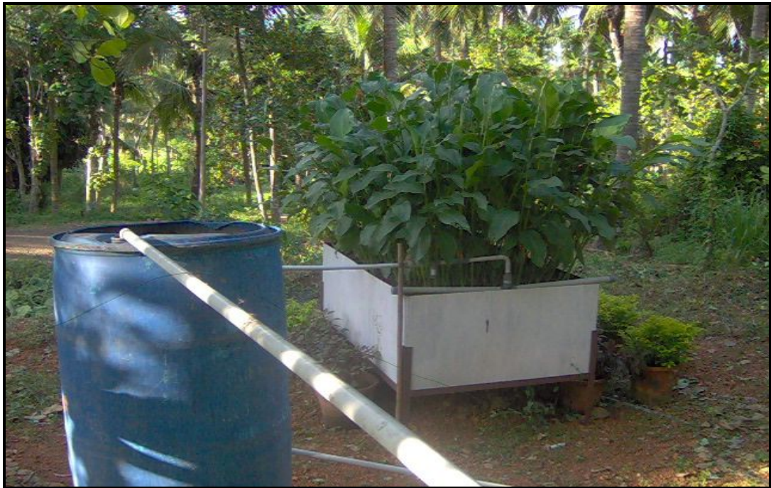
Plate 11 View of SCW system with potted plants and settling tank.
