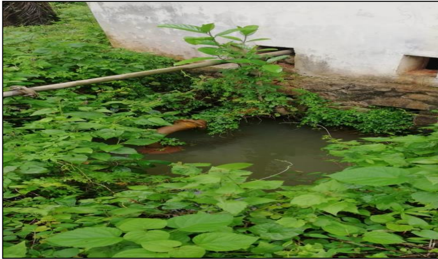
Fig. 3.2 Bore well with a submersible pump in coconut farm: 10.855970 N, 75.984573 E
