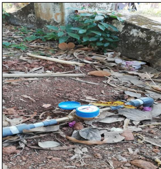
Fig. 3.8 Water Meter at KVK
