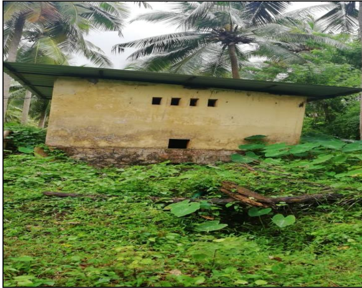
Fig. 3.4 Bore well with centrifugal pump: 10.856203 N, 75.984063 E
