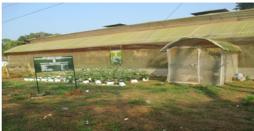
Plate 3.1 Naturally Ventilated Polyhouse
