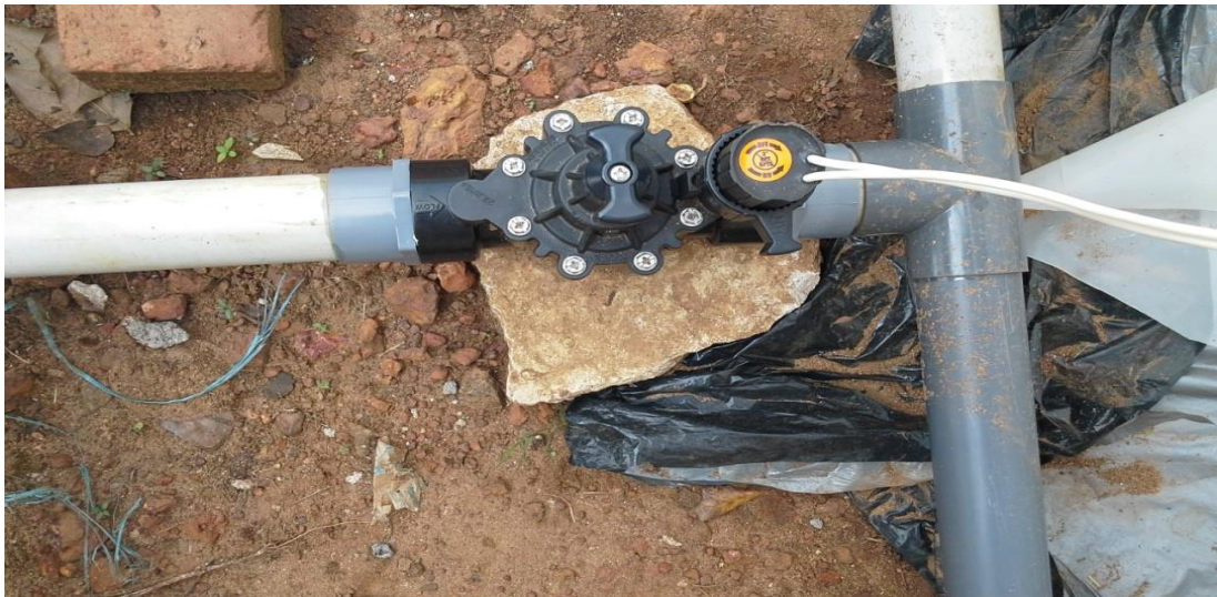
Plate 3.6 Arrangement of solenoid valve
