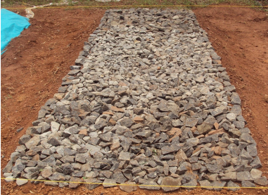
Fig. 3. 6 Road construction using coarse aggregate as the base material
