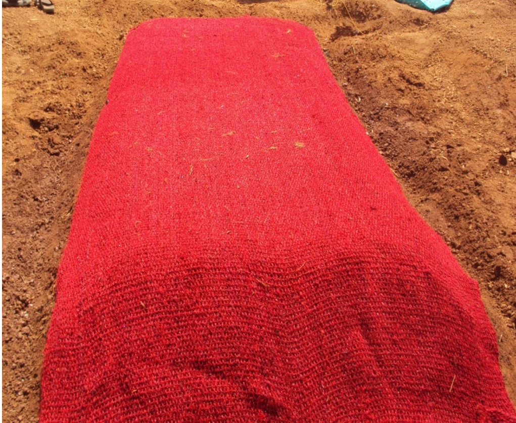
Fig. 3. 3 Road construction using coir geotextile as the base material
