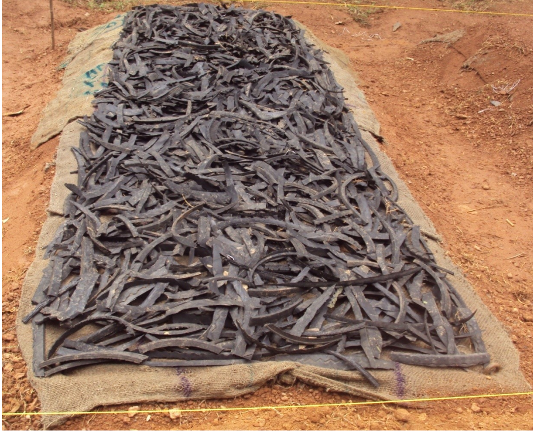
Fig. 3. 5 Road construction using tyre shreds as the base material
