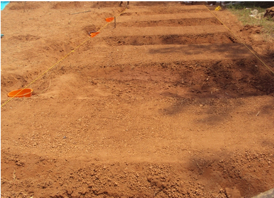
Fig. 3. 2 Road construction using coir geotextile as the base material
