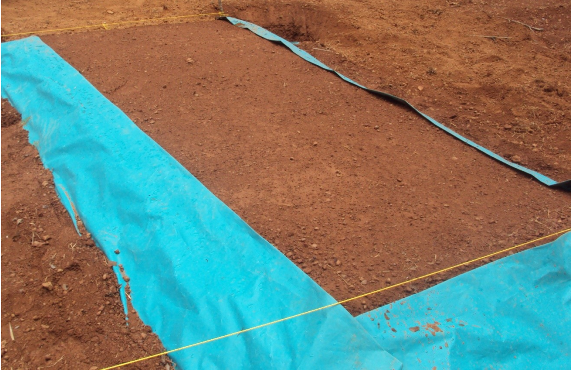
Fig. 3.7 Road construction without any treatment
