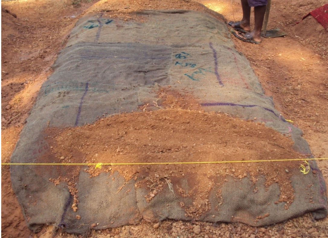
Fig. 3. 4 Road construction using jute as the base material
