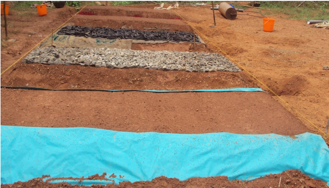
Fig. 3. 8 Five plots of roads reinforced with different materials
