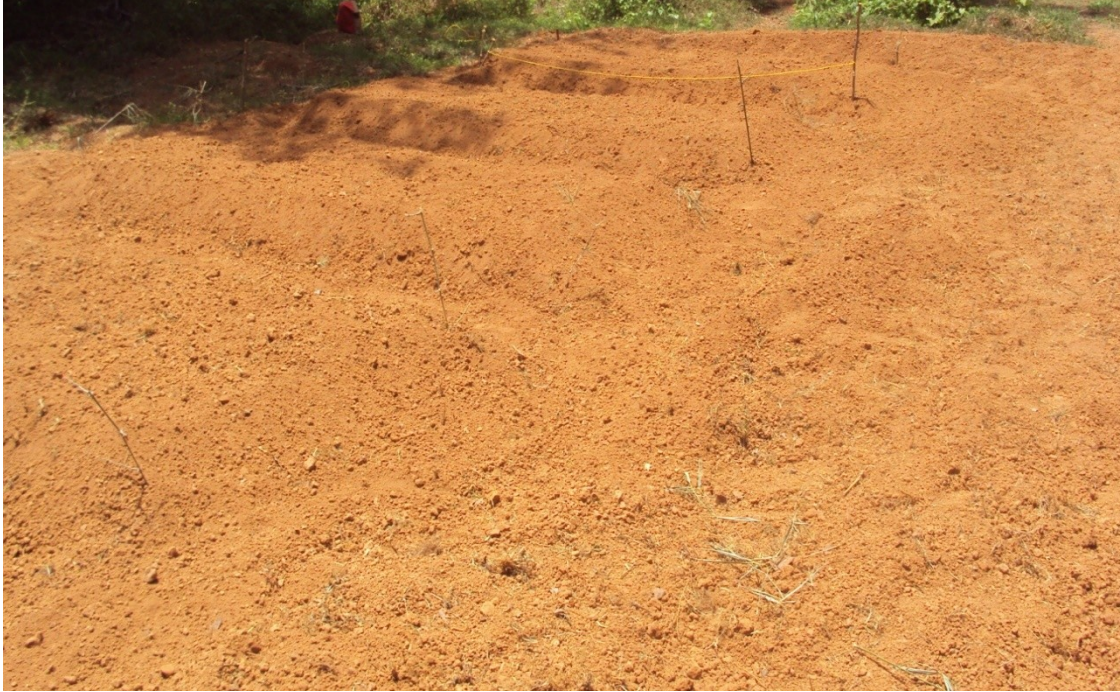
Fig. 3. 1 Site selected for road construction
