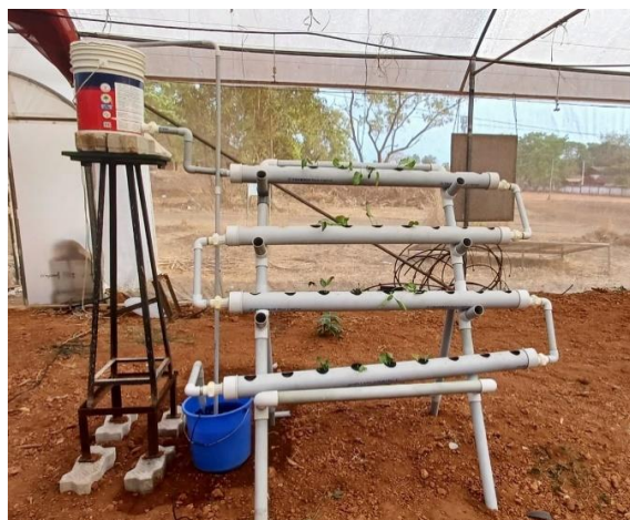
Plate 3.26 Existing hydroponic system
