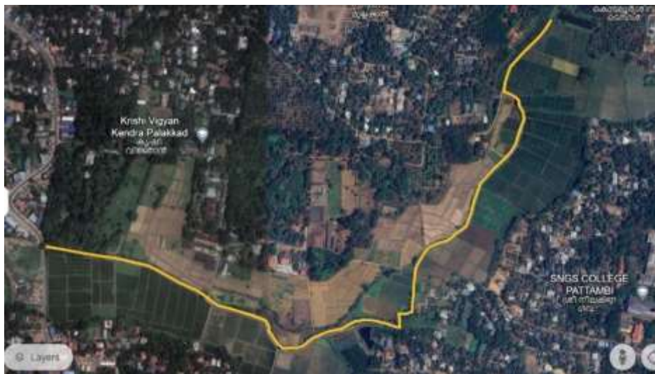
Fig.3.1 Google Earth picture of 1.7 km long canal in RARS Pattambi
