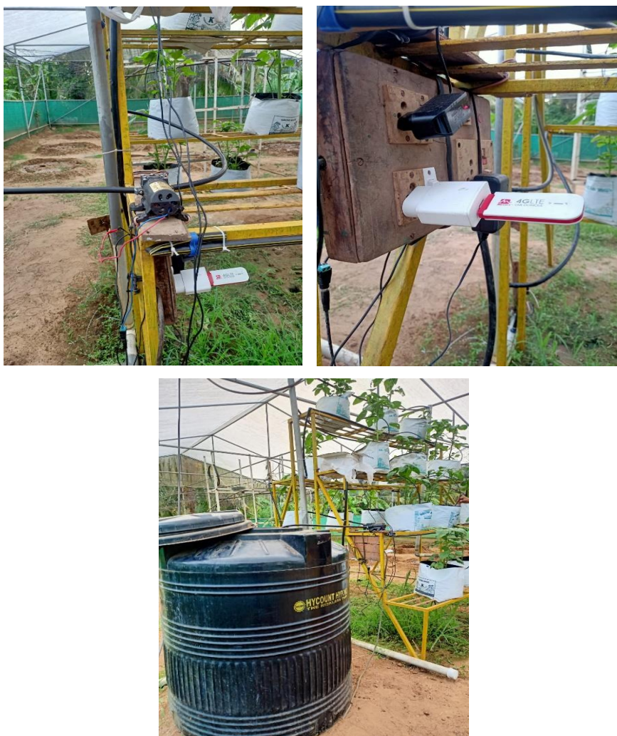
Fig 3.20 Circuit installed in the site
