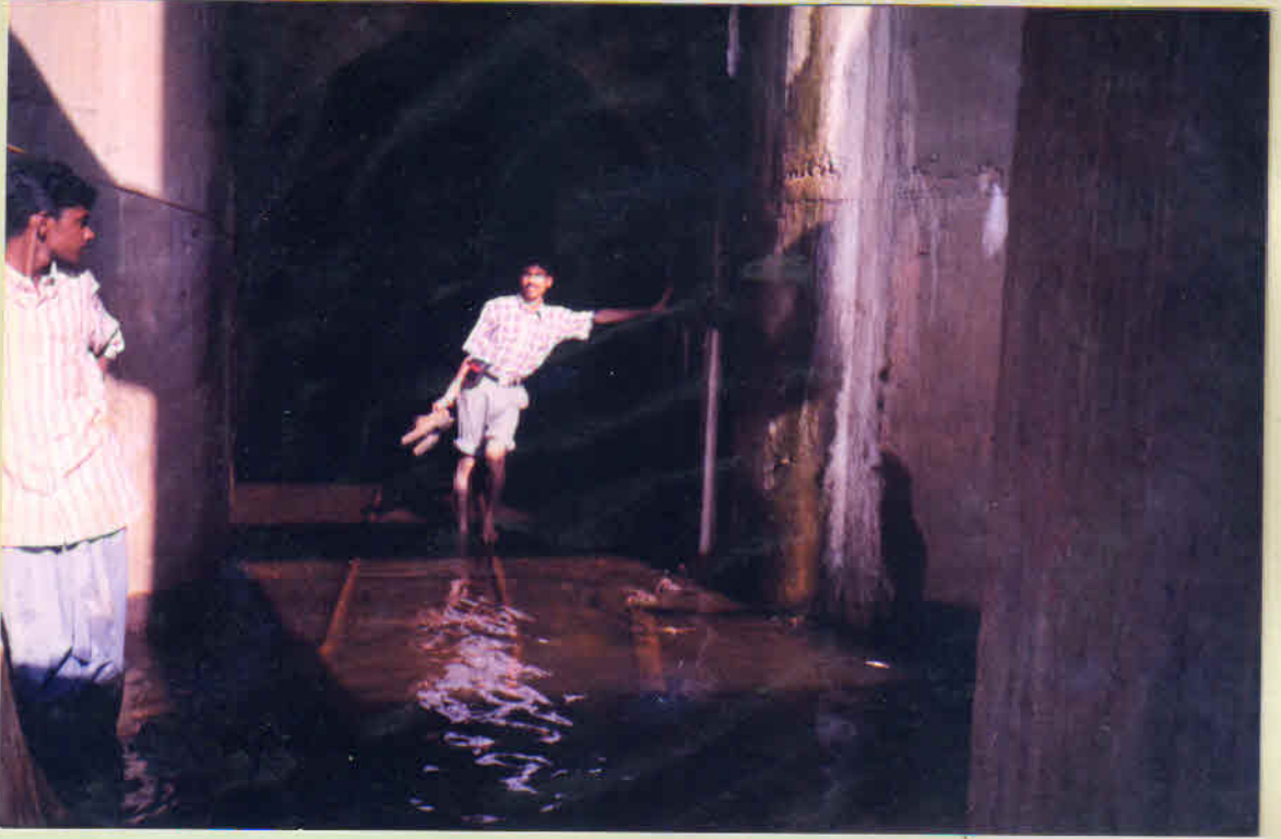
THE TUNNEL CONNECTING VAGAMON CHECKDAM AND IDUKKI RESERVOIR {3.7Km LONG}
