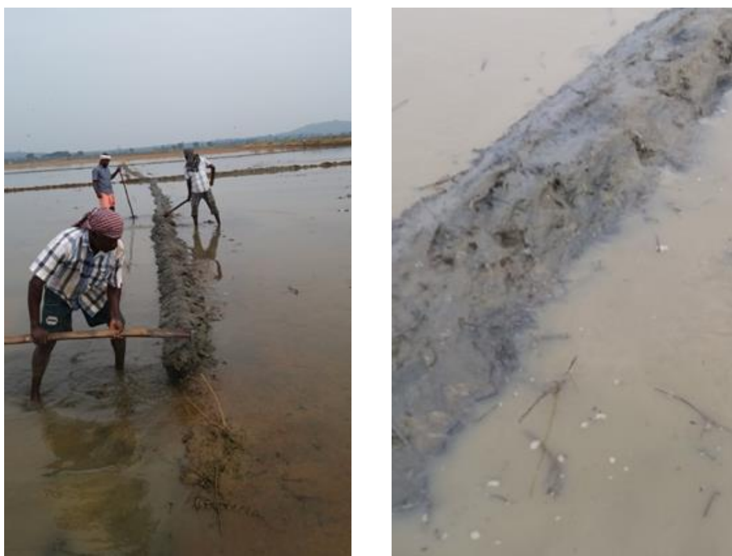
Plate 3.2 Manual strengthening of bunds and formed bund
