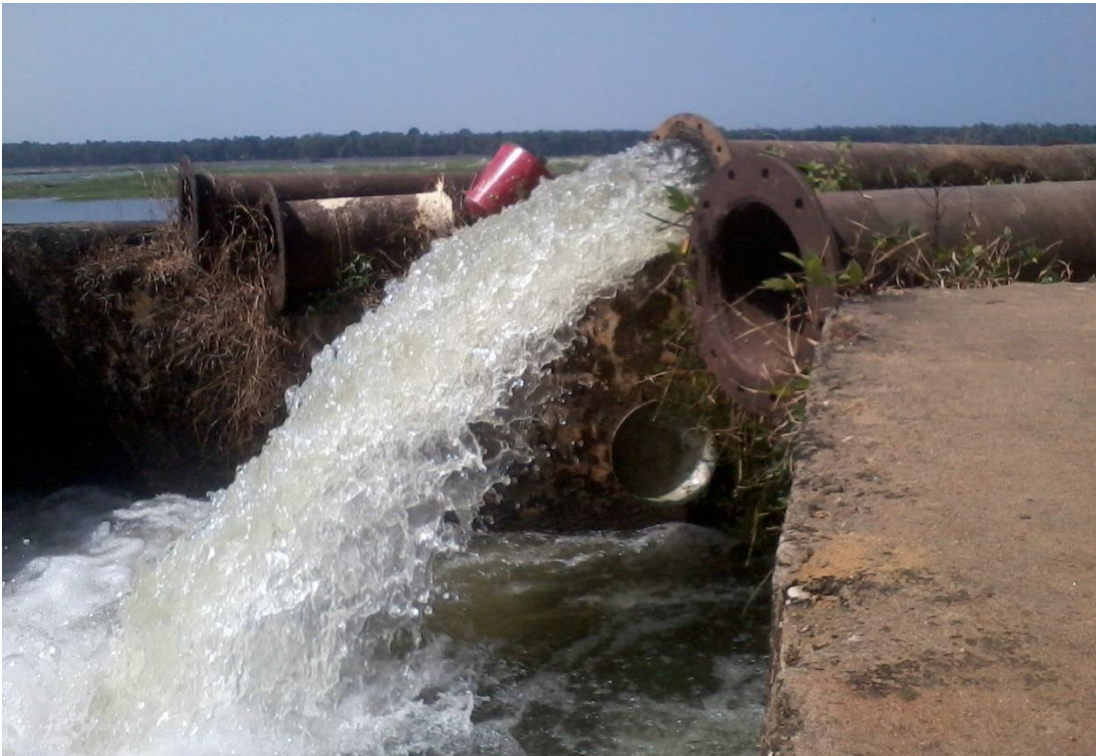
Plate 7. Pumping at Athalur pump house
