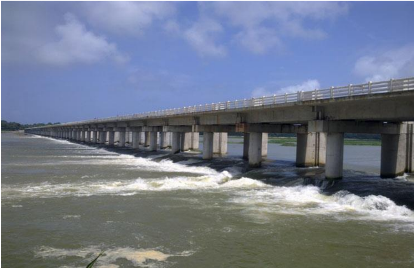
Plate 1. Chamravattom Regulator cum Bridge
