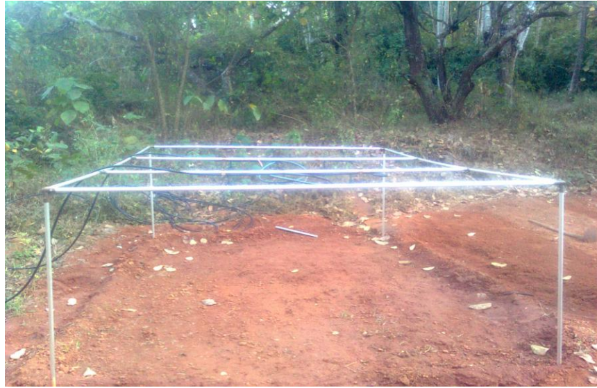
Plate 1: Installation of the supporting frame work in the plot
