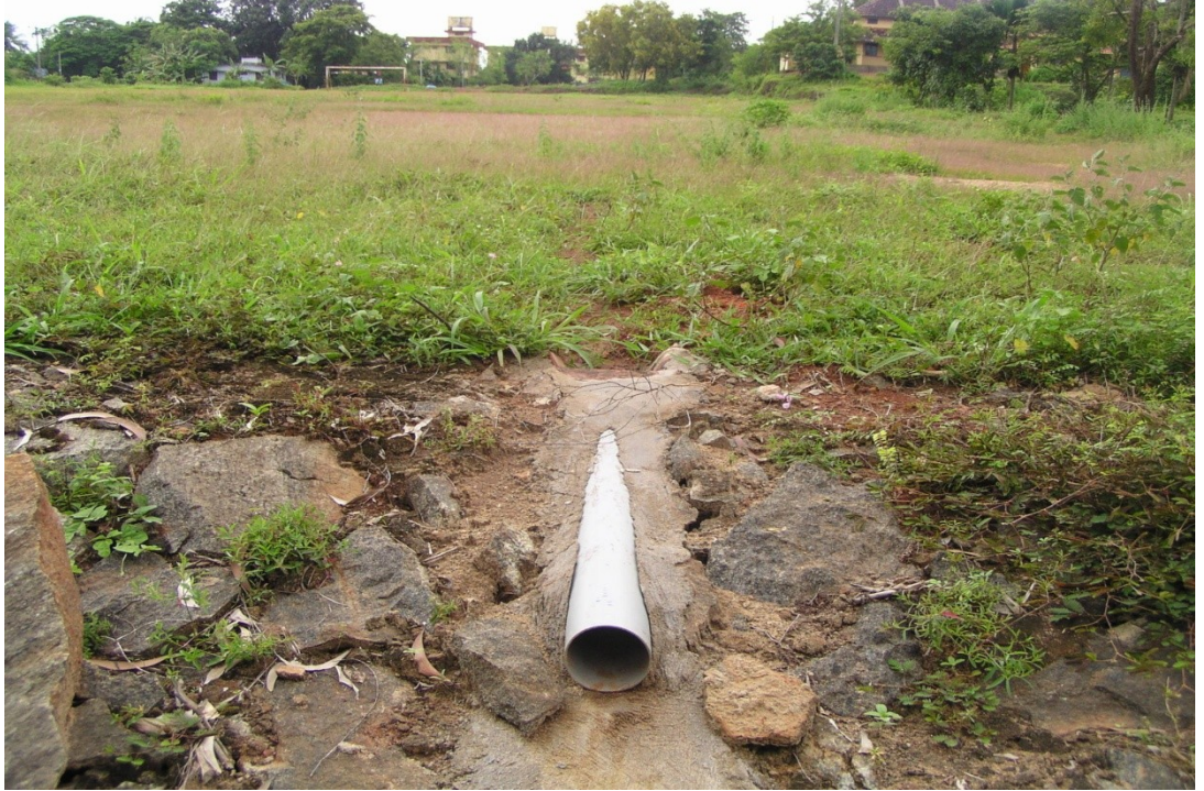
Plate. 8 PVC pipe at the cement plastered area
