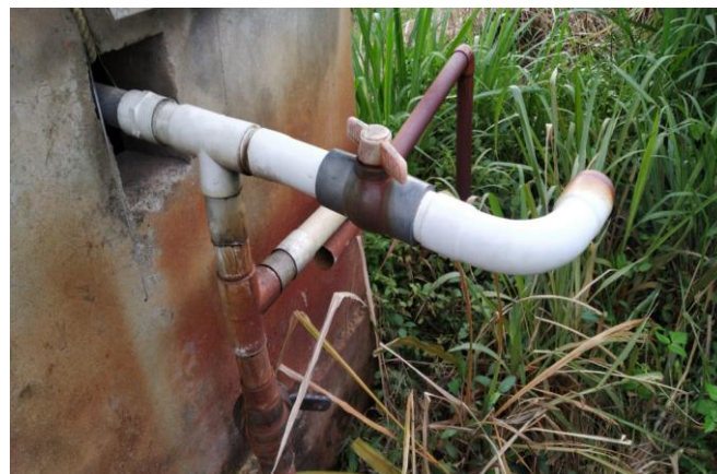
Plate 3.7 Bypass assembly
