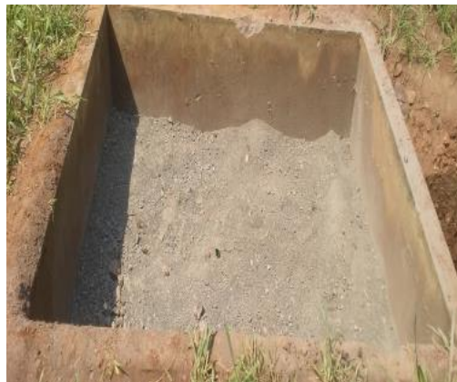
Plate 3.6 Drainage media filling
