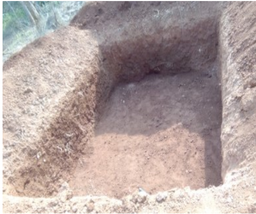
Plate 3.4 Pit for lysimeter installation
