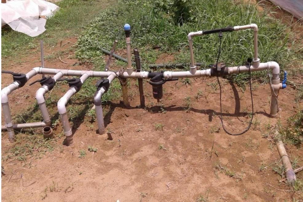
**Plate 3.6 Control system of drip irrigation**
