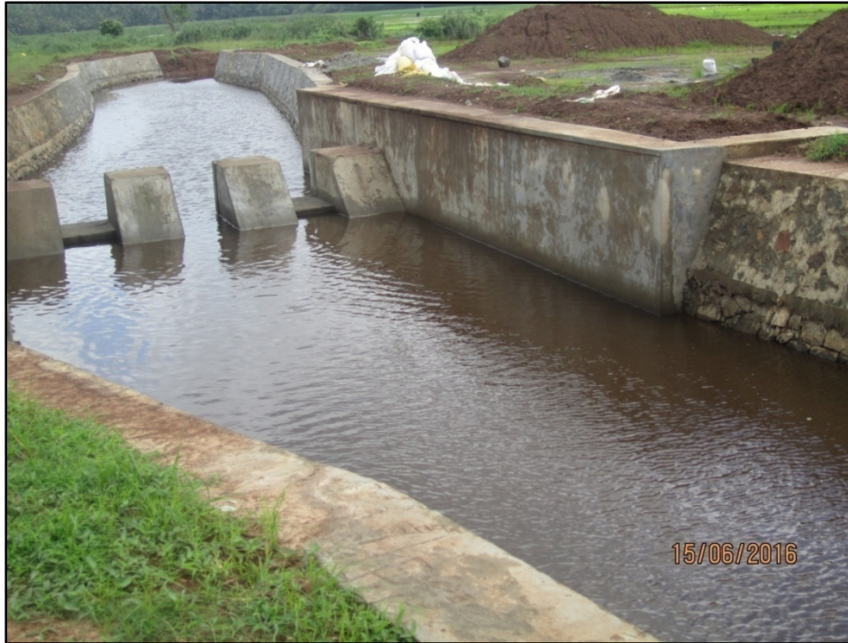
Plate 3 Check dam at Varathurkayal thodu
