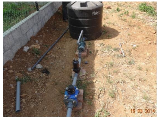
Plate 3.12 Control head components
