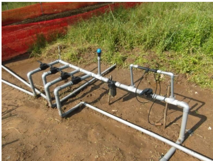
Plate 3.7 Control head of drip irrigation system
