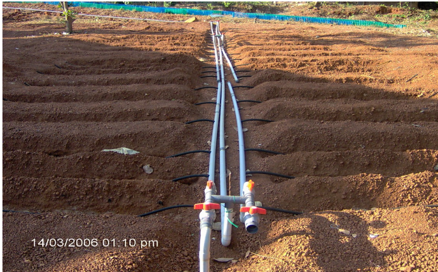
Plate.3.9. .Porous Pipes Installation
