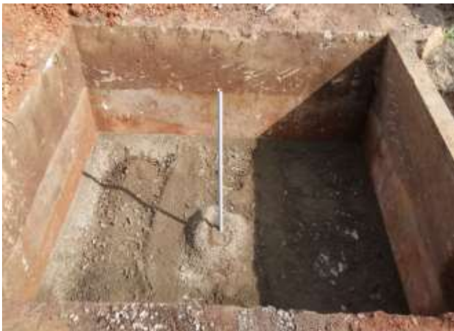
Plate 3.6 Drainage media filling-part 2
