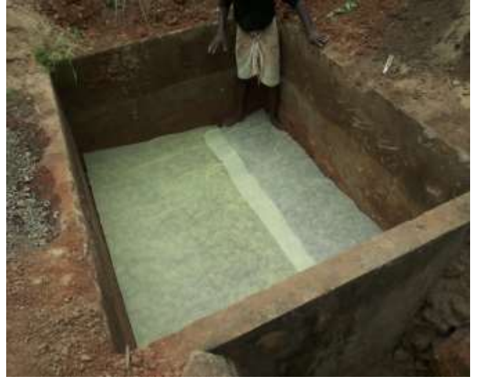
Plate 3.5 Drainage media filling- part 1
