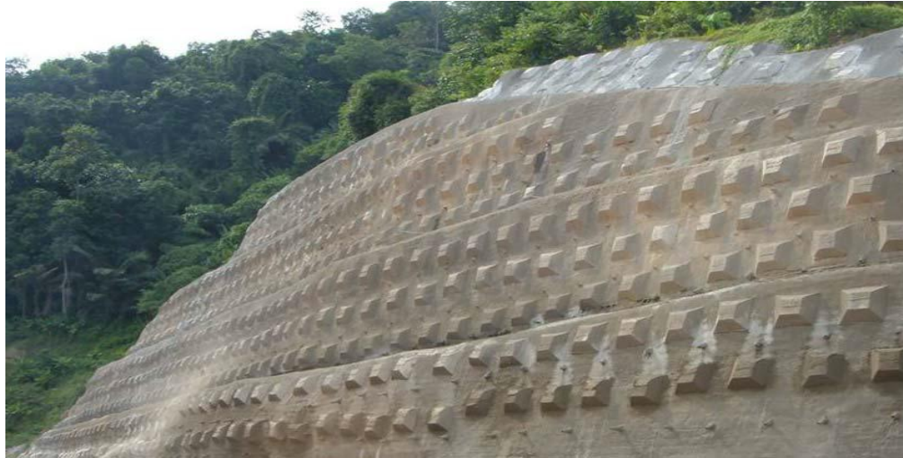
Plate 2.1 20m high soil nailed slope in Kuala Lumpur
