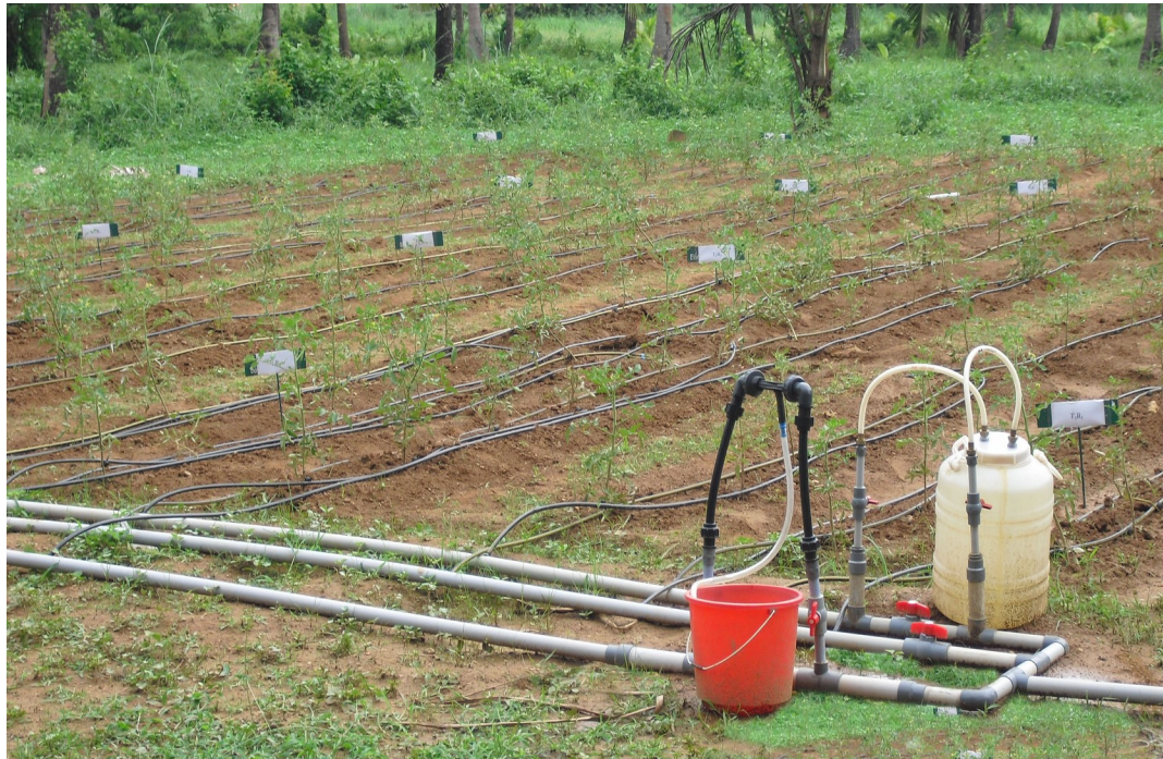
Plate 5 Installation of components of the system
