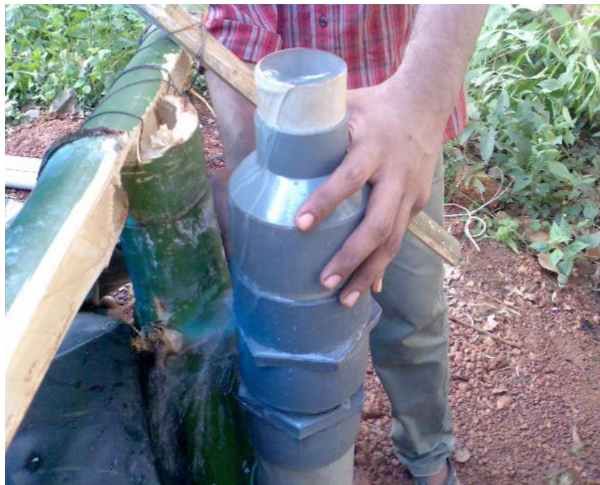
Figure 4.6 Filter unit of the system
