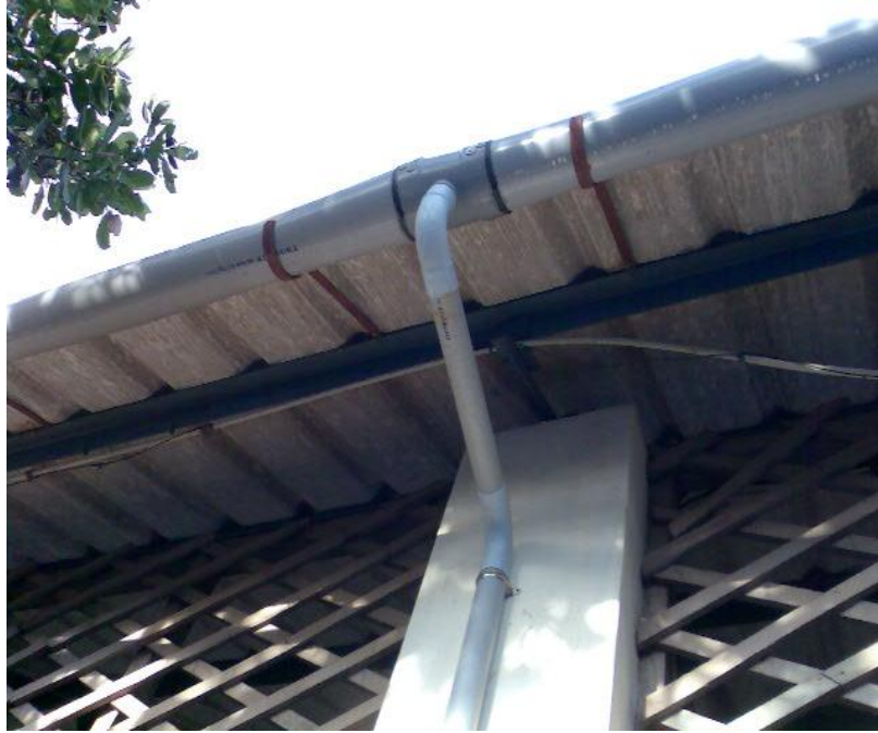
Figure 4.3 Gutter and conveyance system of polylined well
