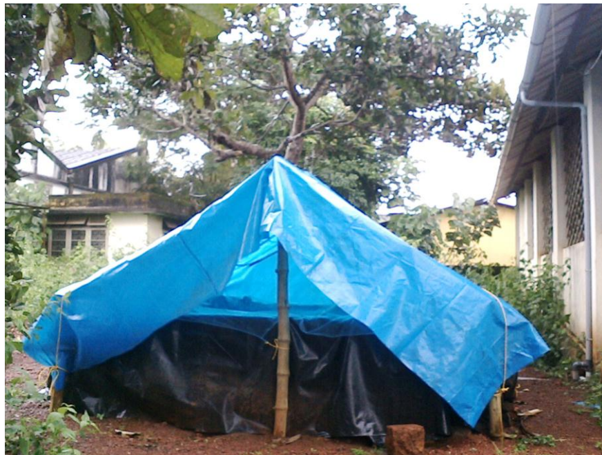
Figure 4.8 Polylined well, 27000 litre capacity
