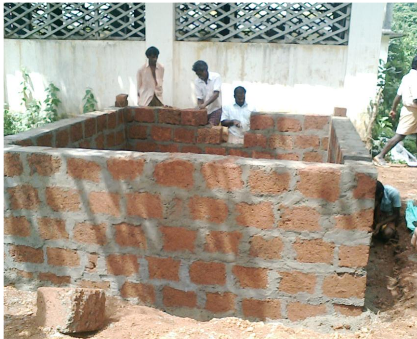
Figure 4.4 Construction of storage tank
