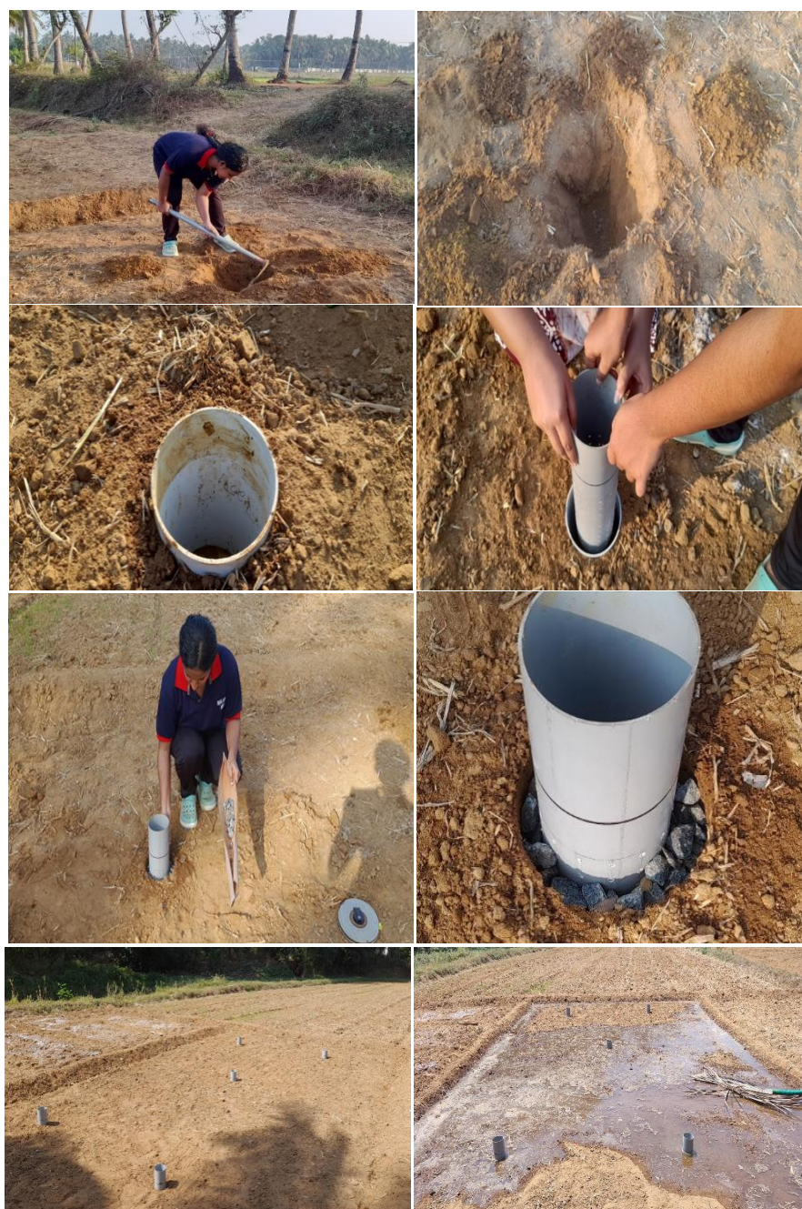
Plate 3.10 Different steps for installation of AWD pipe in field
