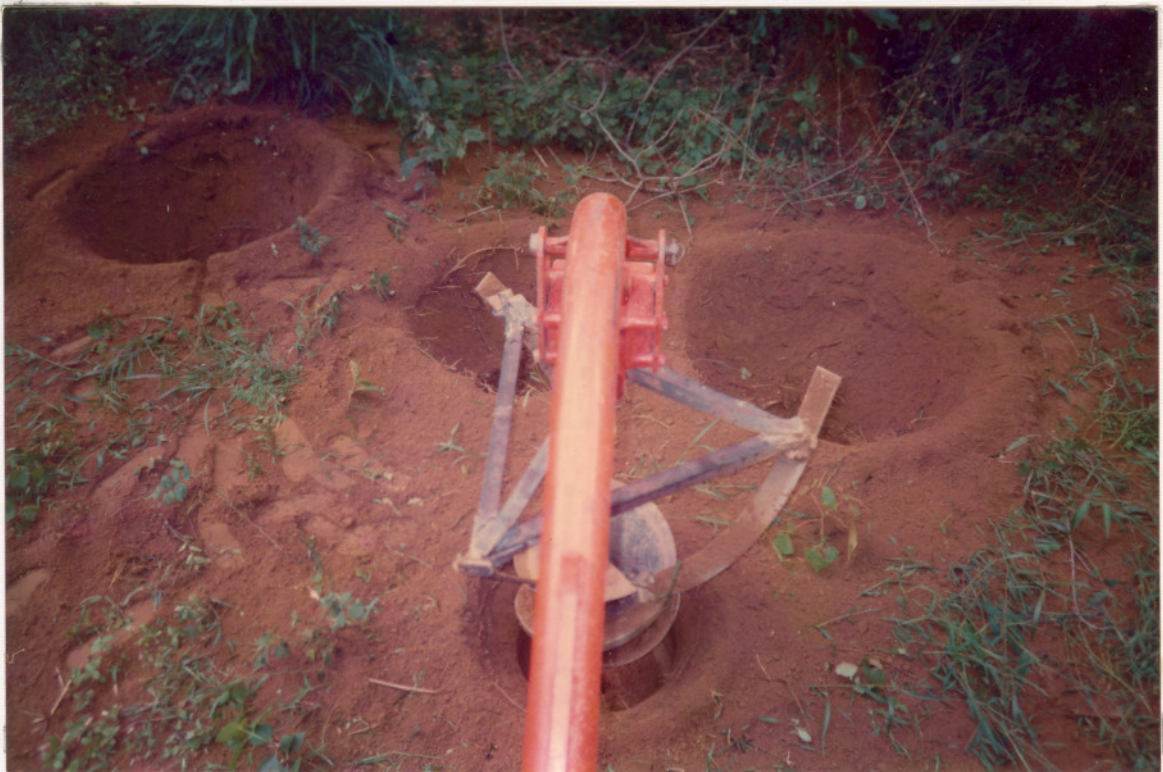
Plate 3.4. Tractor operated post-hole digger with countersinking attachment during field operation (Unit II)
