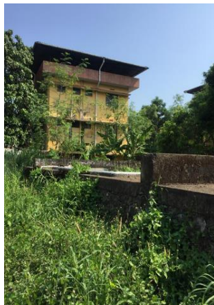
Plate 4.4 Main overhead tank
