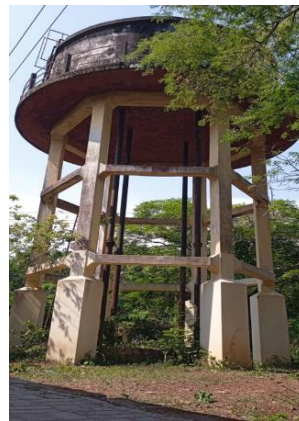
Plate 4.5 Ground level sump
