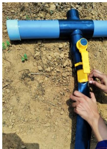
Plate 13. Connecting rainhose to mainline
