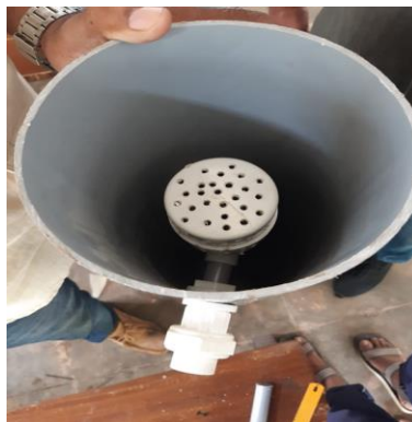
Plate.3.8 Fitting of inlet structure inside PVC casing using tank connector
