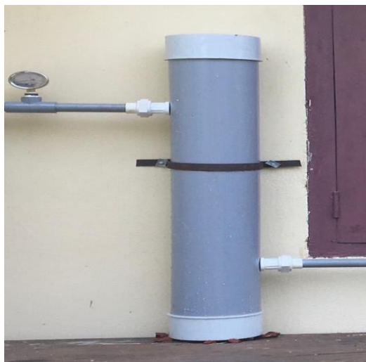
Plate.3.11 Fixing of filter chamber on wall using clamps
