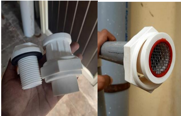
Plate.3.6 Tank connector with strainer
