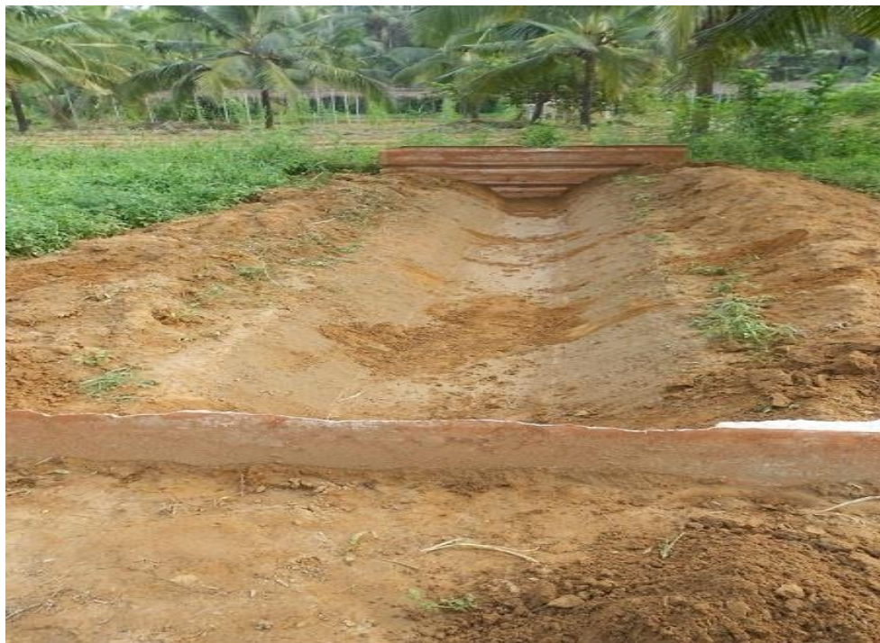
Plate 4: Control channel before ponding
