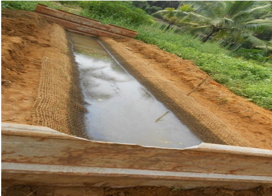
Plate 5: Coir Geo-textile lined channel at the time of ponding
