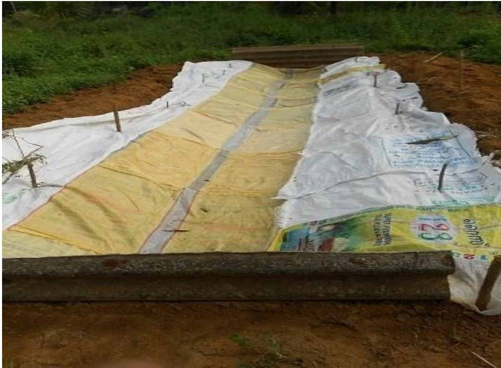
Plate 3: Plastic sheet material lined channel before ponding
