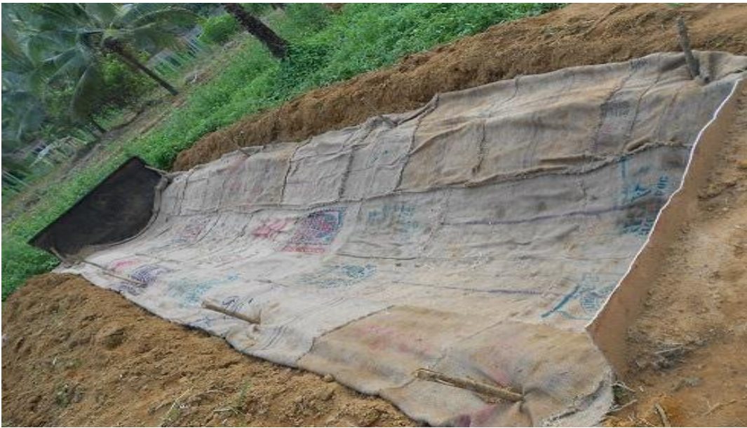
Plate 2: Gunny cloth lined channel before ponding
