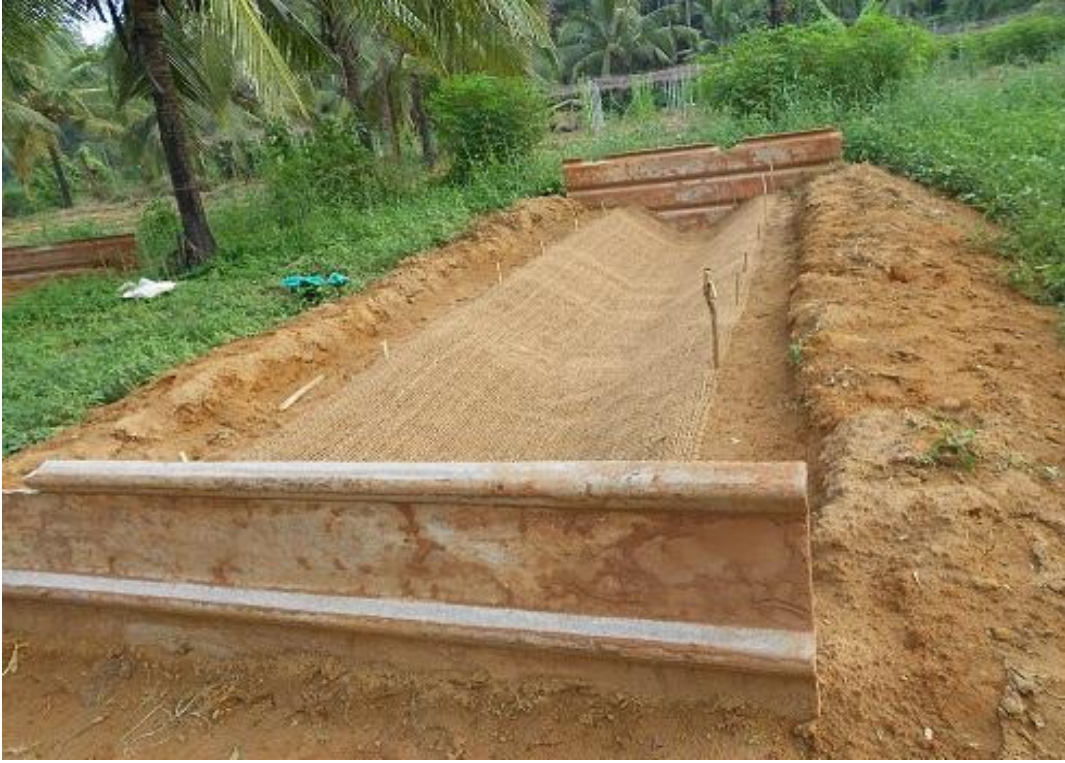
Plate 1: Coir Geo-textile lined channel before ponding
