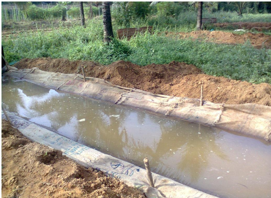
Plate 6: Gunny cloth lined channel at the time of ponding
