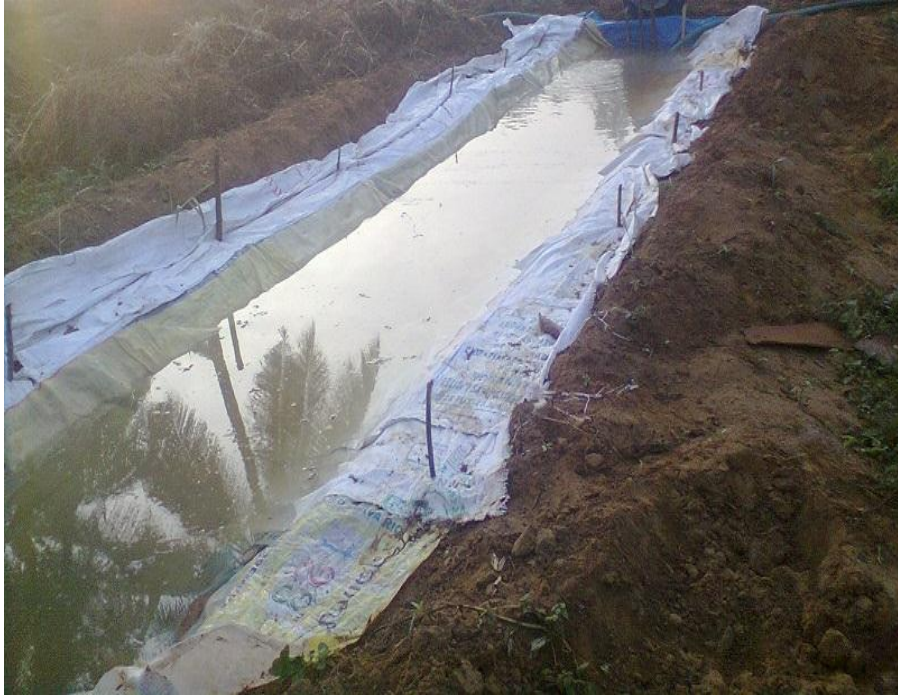
Plate 7: Plastic sheet lined channel at the time of ponding
