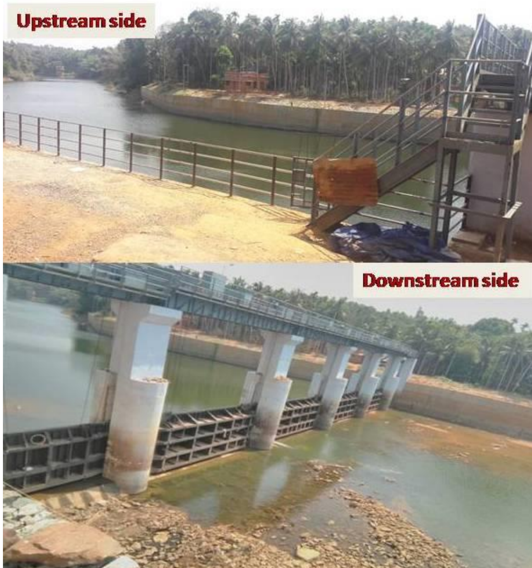
Plate 1. Upstream and Downstream side of Bakkikayam Regulator
